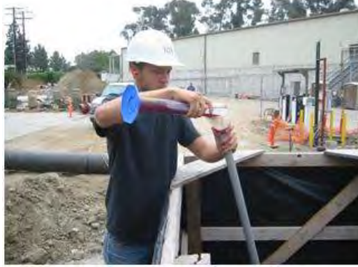
Figure 2: Injection of Rhodamine WT Dye into CCT Influent Box at LAWRP
