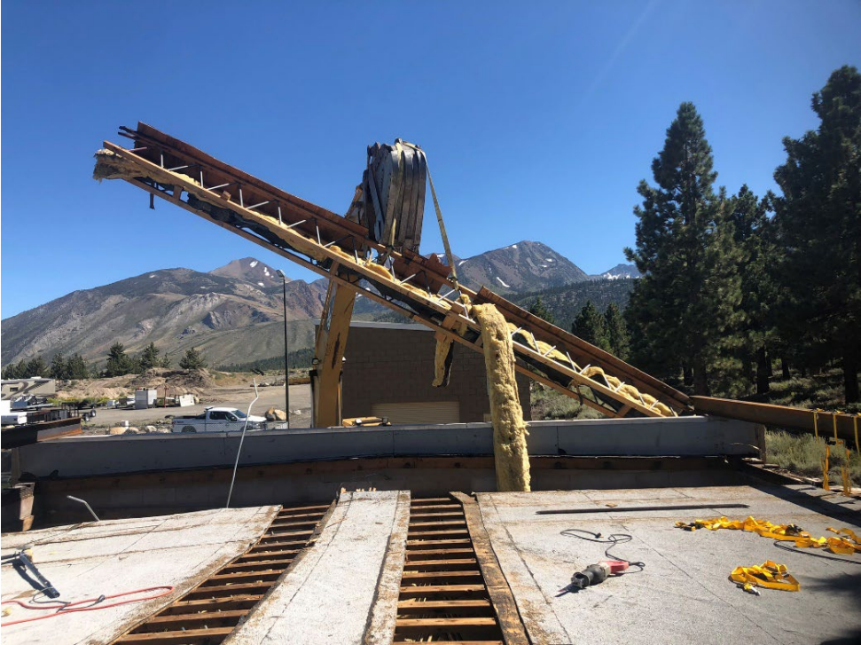
4- Removal of Trusses
