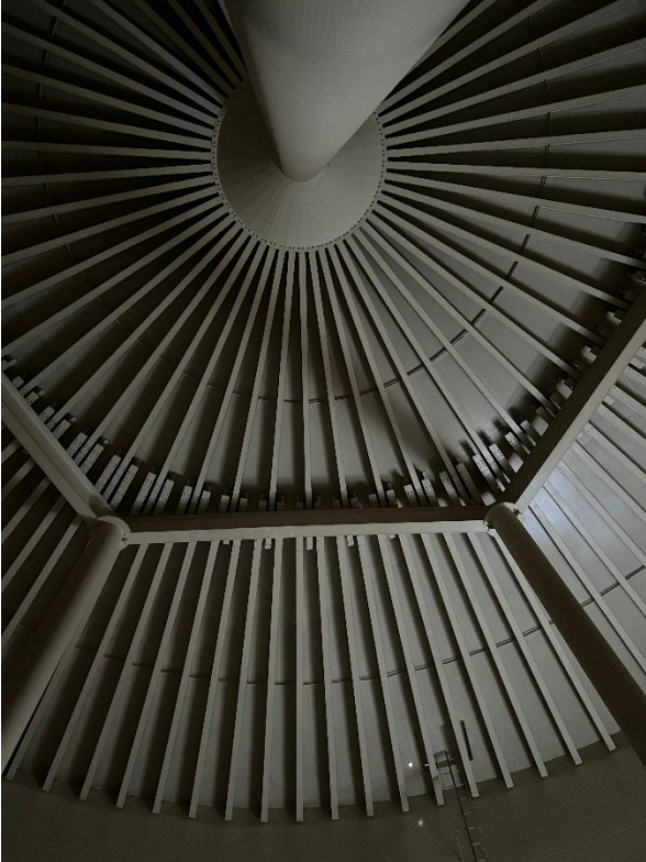
5- Completed Interior Structure
