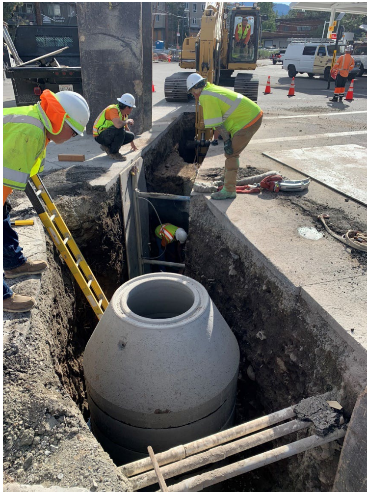
5- Constructing New Manhole
