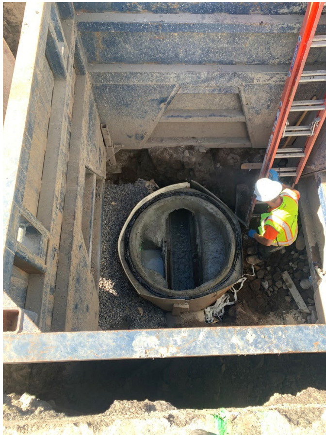
3- Constructing New Manhole Base
