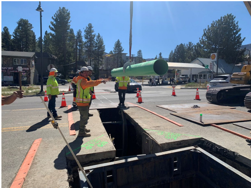
4- Laying New 15" Sewer Pipe
