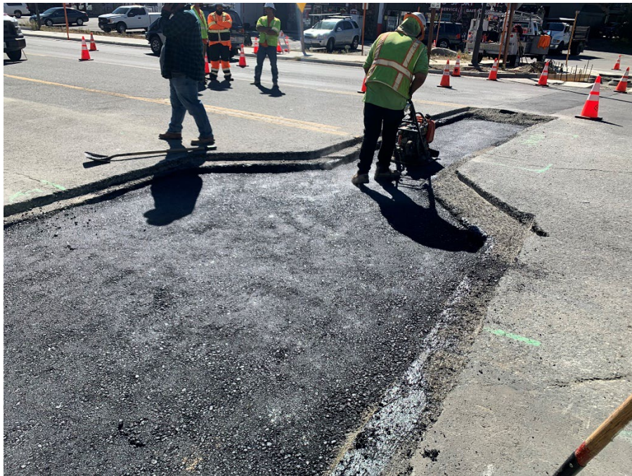
6- T-Patch Trench Paving
