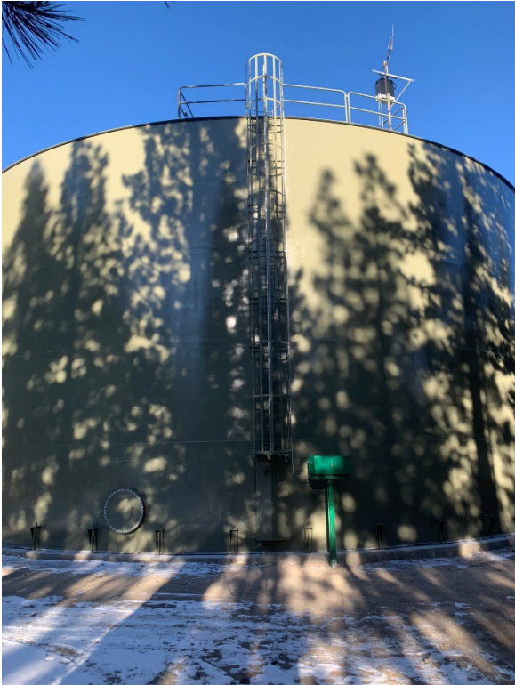
6- Completed Tank Exterior and Manway
