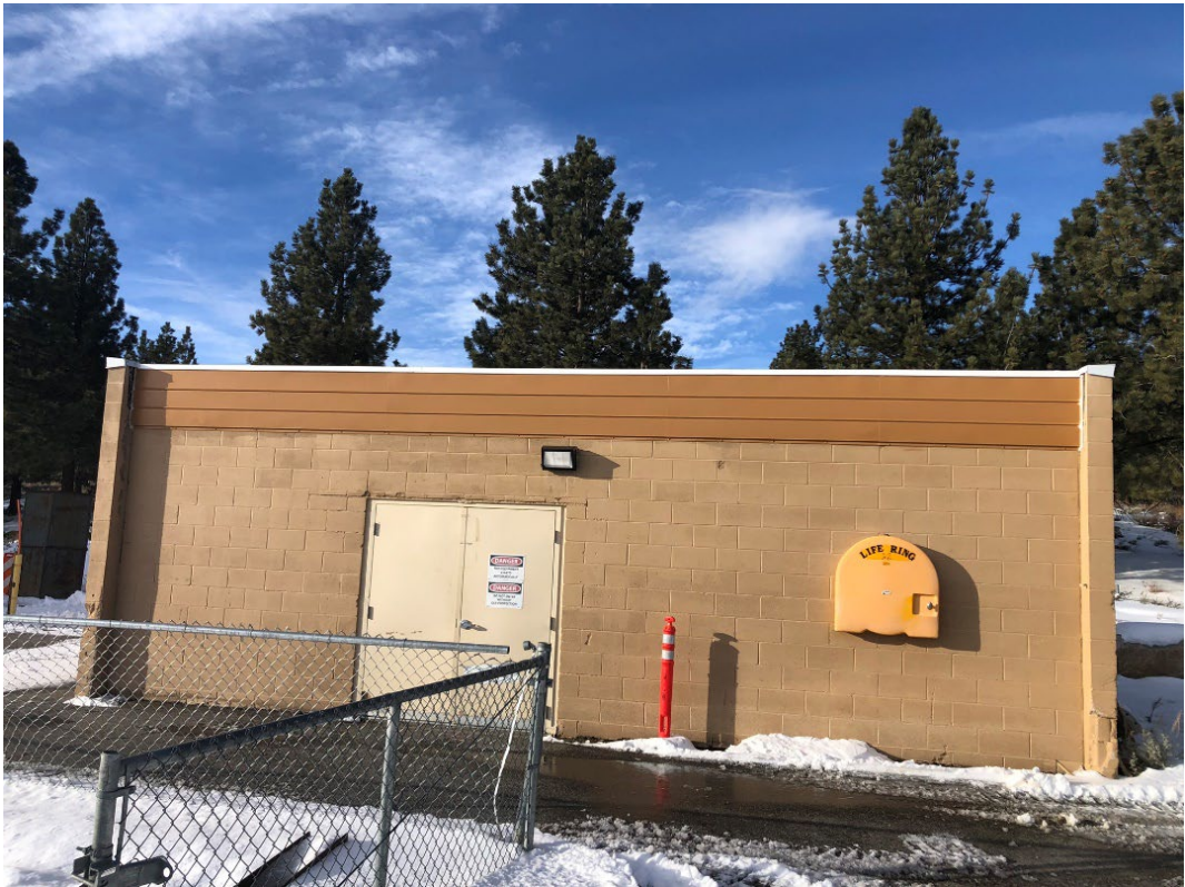
8- Front of Building
