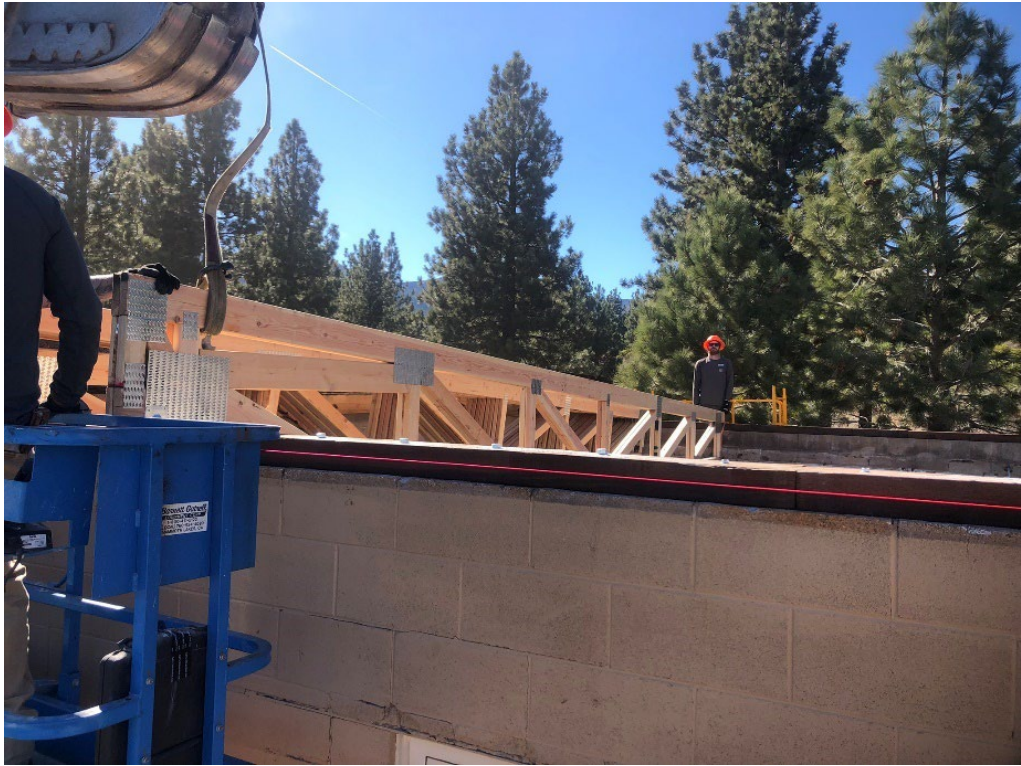
5- Sloped Truss Profile
